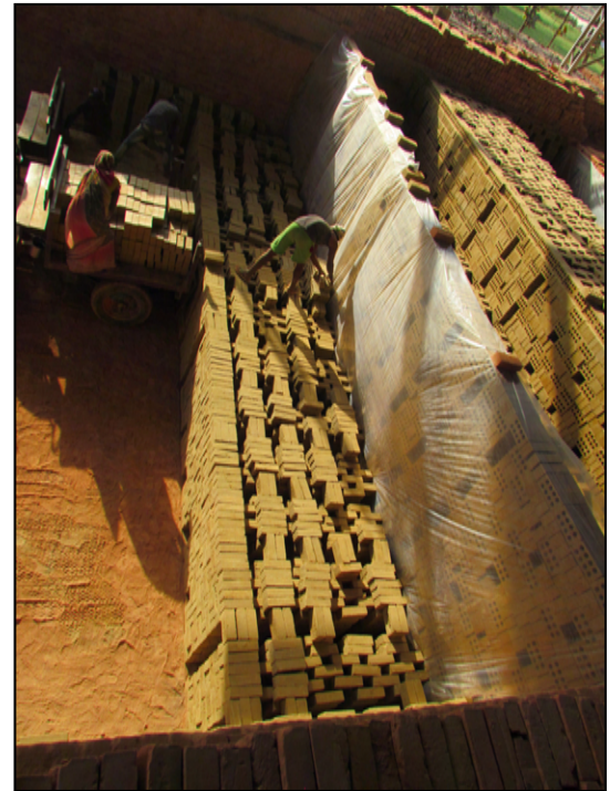
Figure 4.15: Putting plastic sheet on the last row of chamber
