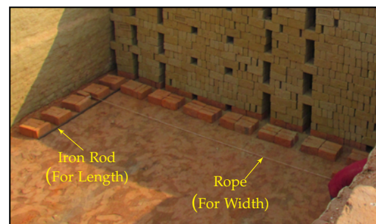
Figure 4.6: Bottom course of chamber
