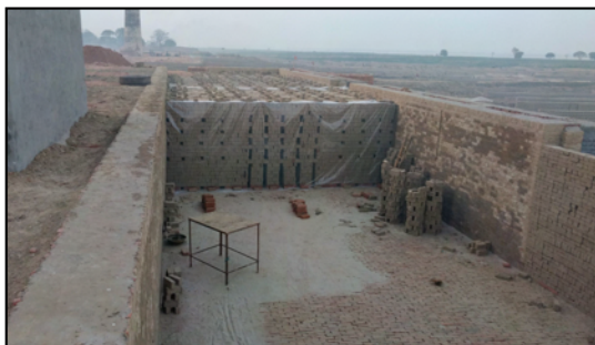
Figure 4.3: Kiln floor laid with fired-bricks
