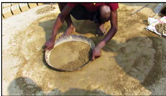
Figure 2.2: Levelling of moulding area
