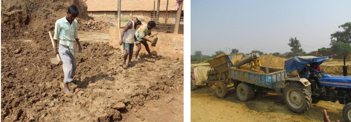
Figure 8: Soil mix preparation – Manually and by pug-mill
