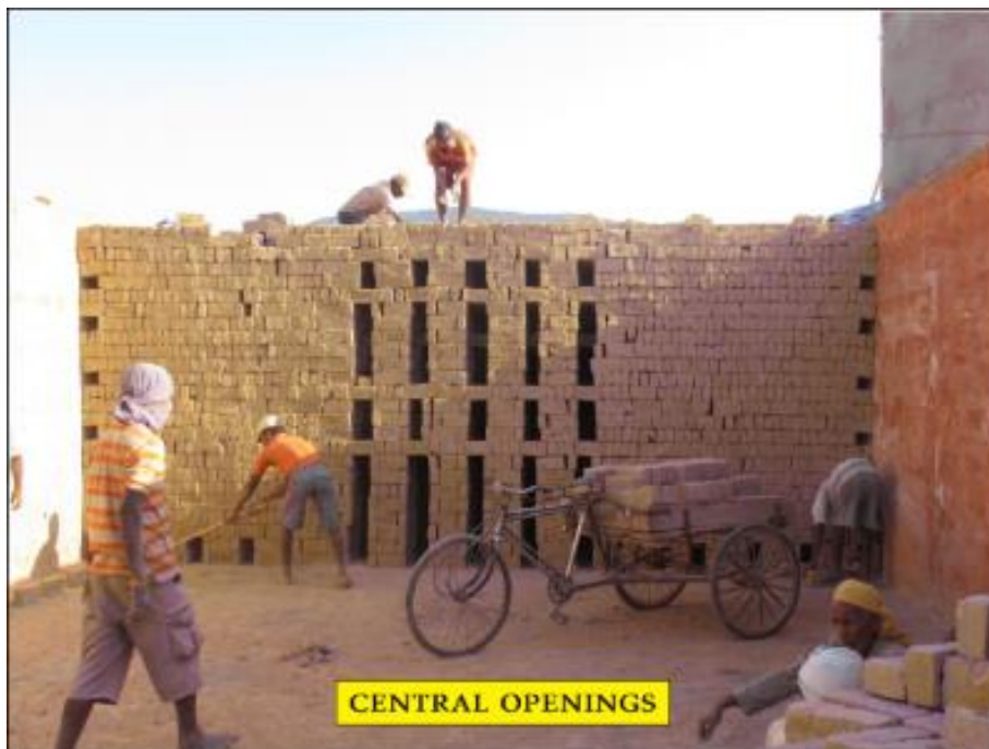
Figure 87: Openings at the middle of a chamber
