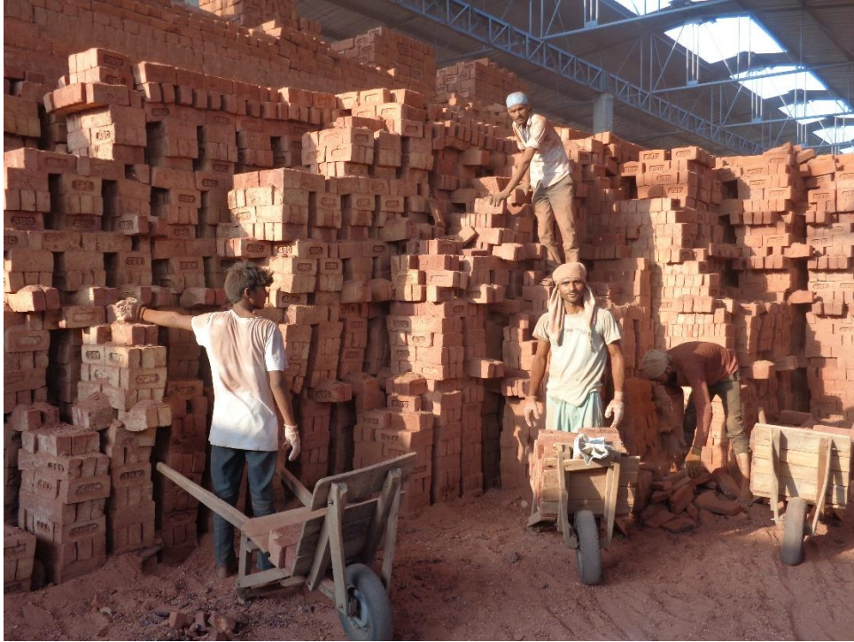
Figure 31: Unloading of bricks
