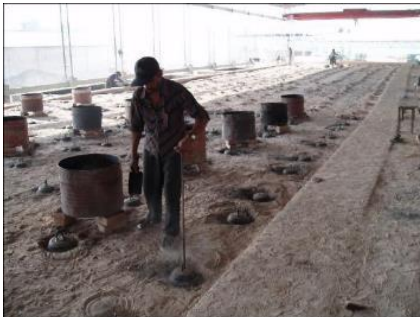
Figure 91: Single fireman feeding fuel in a Zig-zag kiln
