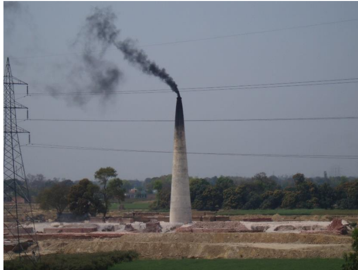
Figure 73: Fixed chimney Bull's trench kiln
