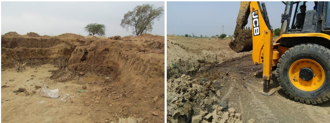
Figure 7: Soil Winning – Manual or by excavator
