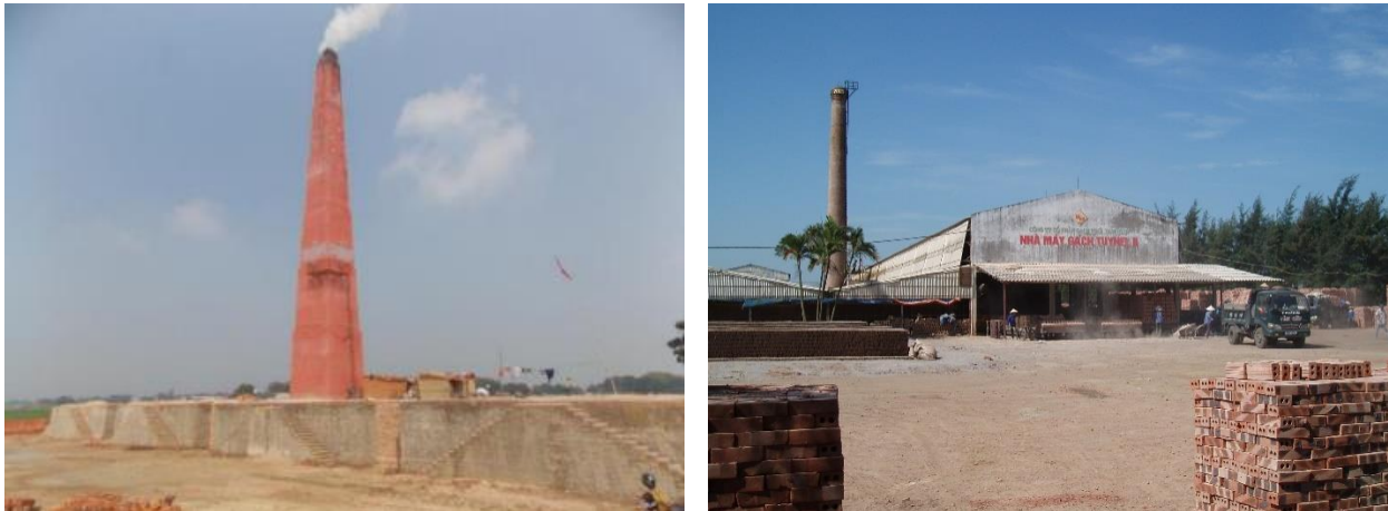
Figure 19: Zigzag Kiln and Tunnel Kiln
